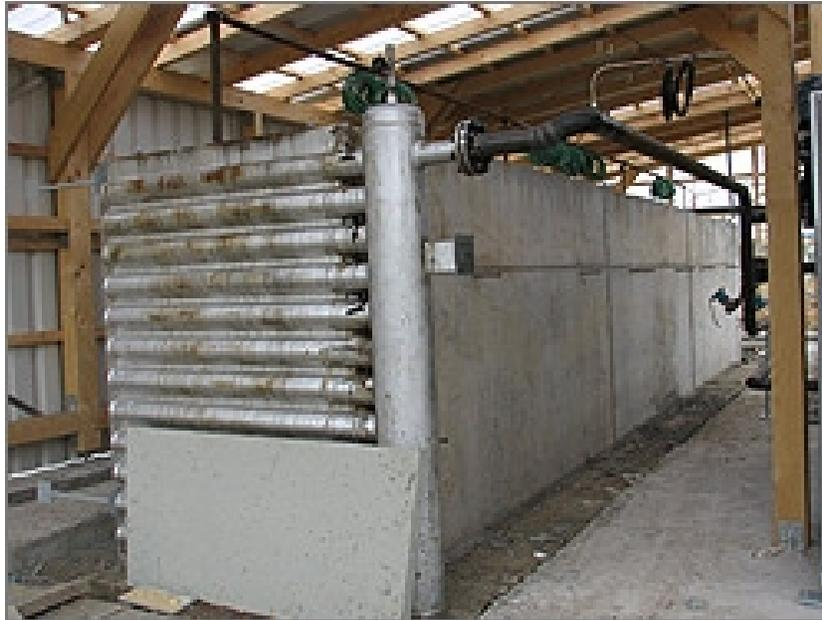
Figure 2. Concrete thermal energy storage unit.
