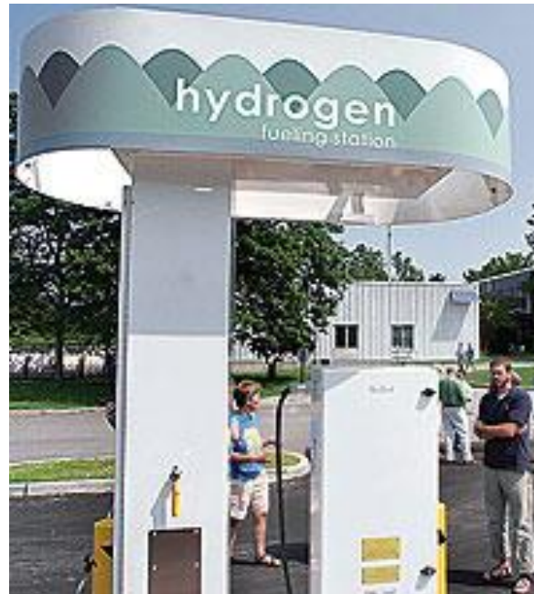
Figure 1. Hydrogen automobile fuel cell refueling station at Burlington, Vermont. Electrolysis is used to dissociate water into hydrogen and oxygen. Source: USDOE.
