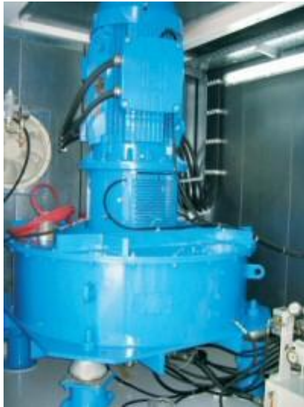
Figure 3. Enercon 200 kW of rated power and 5 kW.hr of energy storage capacity flywheel for use with a standalone wind power system. Source: Enercon.
