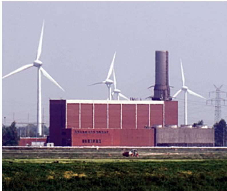
Figure 3. A 290 MW Compressed Air Energy Storage (CAES) in conjunction with wind power at Huntorf, Germany [2].
