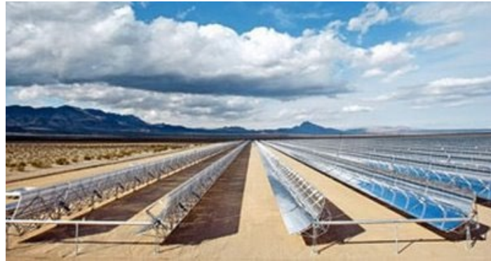
Figure 33. Solar 3 parabolic trough collector plant.
