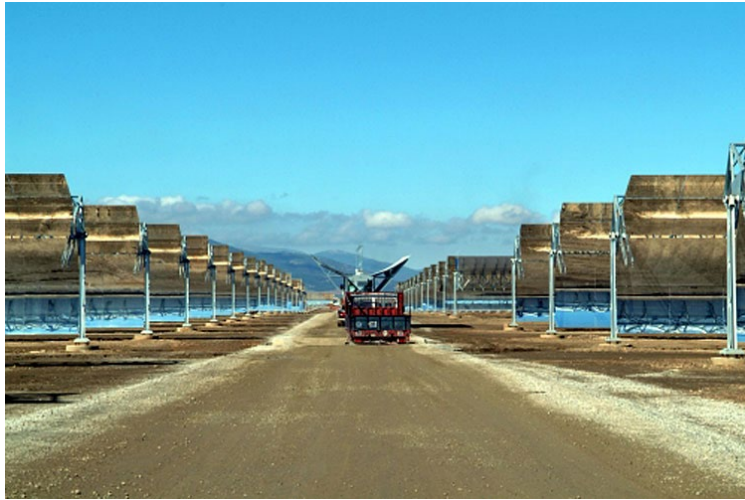
Figure 36. Andasol 1 plant, Solar Millenium, Spain.
