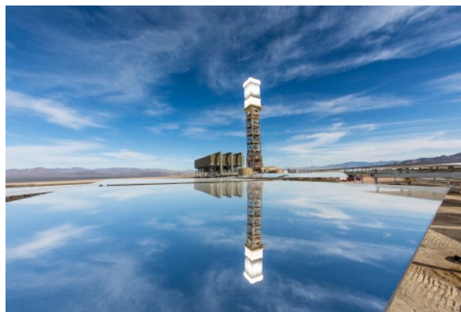
Figure 42. Tower number 1 at the Ivanpah plant, height =459 ft.
