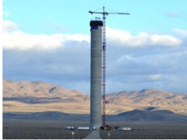
Figure 50. Solar reserve Crescent Dunes 110 MW, Tonopah, Nevada solar plant uses 10,000 billboard-size mirrors and thermal energy storage in a molten salt.
