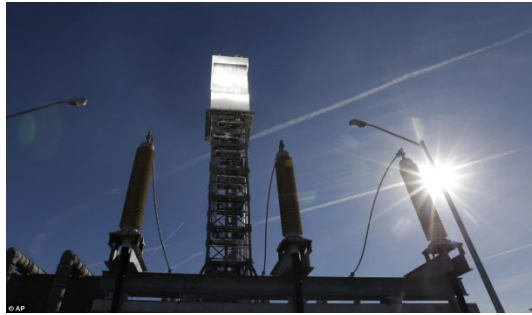
Figure 48. Boilers of the Ivanpah plant. Owned by NRG Energy, Google and BrightSource Energy. Plant does not use energy storage, but steam is used for the secondary recovery of oil by the Chevron oil Company.
