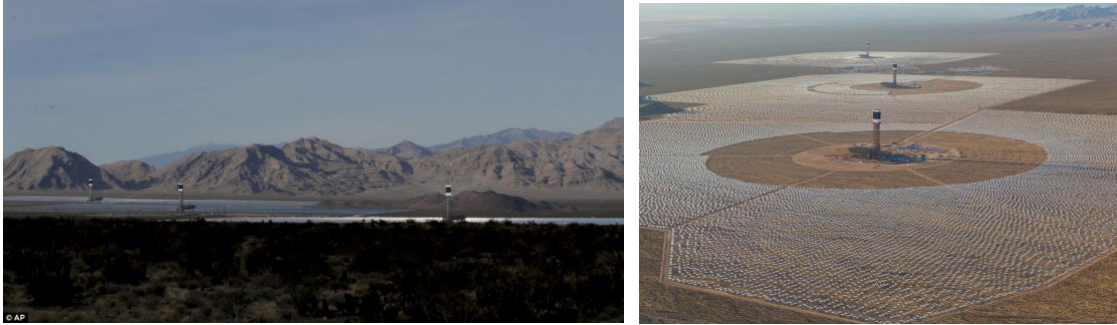
Figure 40. Ivanpah power plant consists of three towers at the Ivanpah dry lake.
