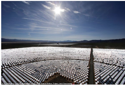
Figure 44. Ivanpah 300,000 flat mirrors array.
