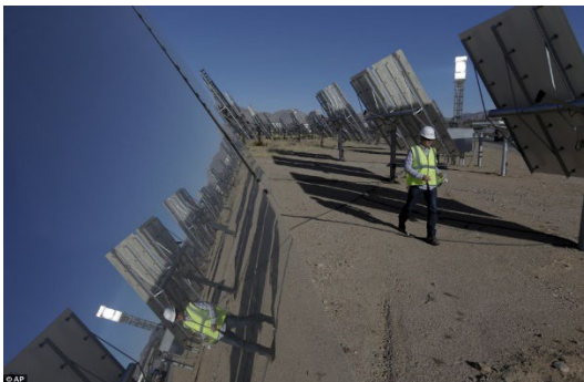
Figure 44. Ivanpah 300,000 flat mirrors array.
