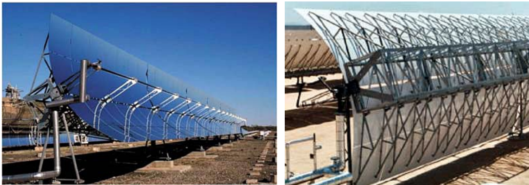
Figure 29. Front and back views of parabolic trough Skal-Et 150 at Al Kuraymat, Egypt, 2010. Peak optical efficiency: 80 percent. Geometric concentration: 82. Length: 123.75 m / SCA. Aperture area: 817.5 m 2 /SCA [16].
