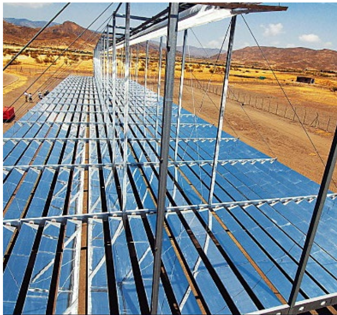
Figure 37. Plataforma Solar Fresnel concentrating plant, Almeria, Spain.
