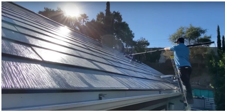
Figure 9. Water washing the surface of Barium titanate crystal film solar cells.
