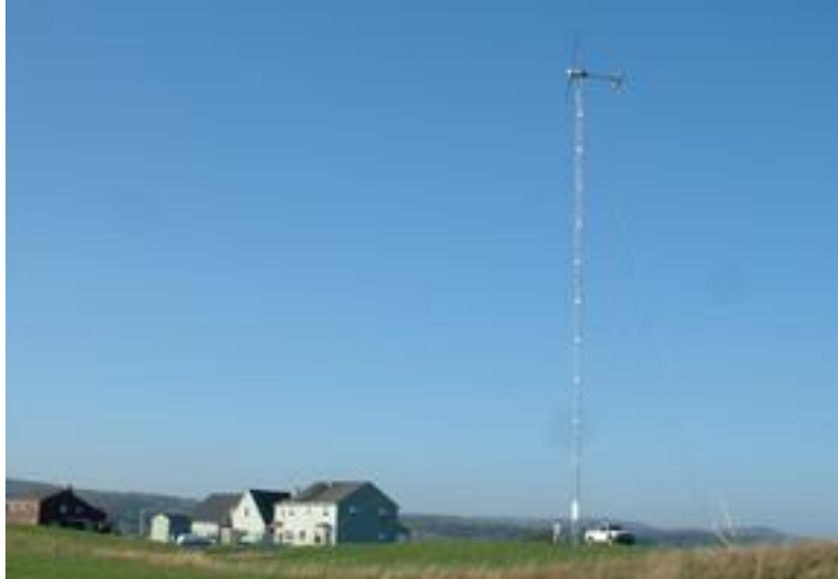
Figure 2. A 10 kW wind turbine on a 120 foot tower with guy-wires in a rural environment can provide the electrical needs for a typical USA household with energy storage.
