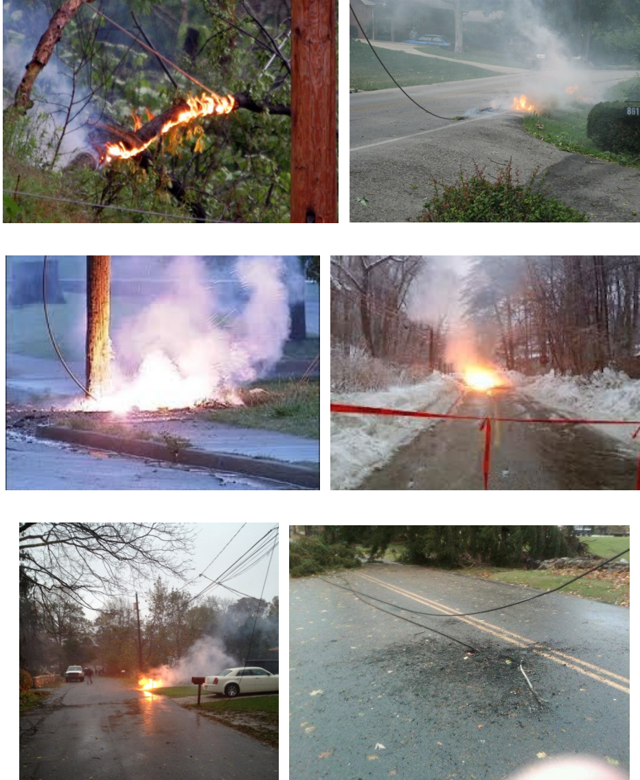
Figure 44. Downed overhead power lines constitute a fire hazard in addition to their electrocution hazard.
