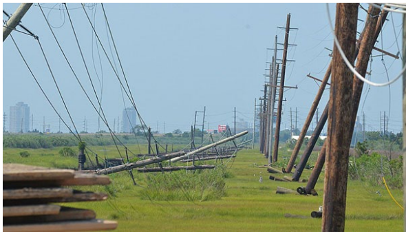
Figure 43. Downed overhead power lines in the open countryside cause widespread power failures in both rural and urban sites.
