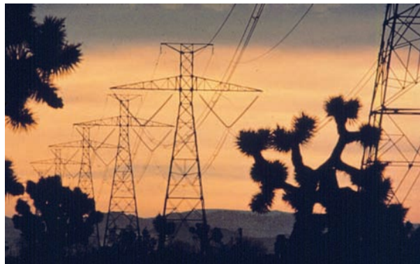
Figure 30. Overhead 500 kV lines use only two conductors in HVDC, compared with 3 conductors in HVAC. Overhead lines can be used in low-population areas. Source: IEEE.
