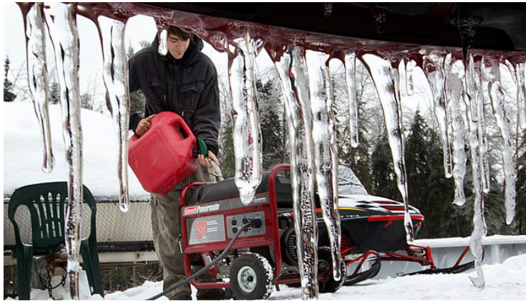
Figure 50. Running electrical emergency generator in power outage presents CO toxicity and electrocution hazards under wet conditions. Bowdoin, Maine, USA December 26, 2014.
