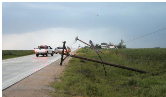
Figure 43. Downed overhead power lines in the open countryside cause widespread power failures in both rural and urban sites.
