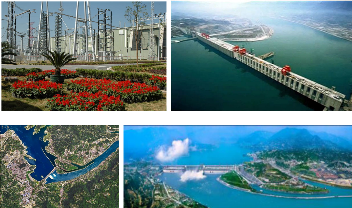
Figure 1. Modern state-of-the-art Yidu High Voltage Direct Current (HVDC) converter station serves the 22,500 MW world's largest hydroelectric power station Three Gorges Dam on the Yangtze River, 403 square miles reservoir project at Shanghai, China. The dam became fully functional on July 4, 2012. Source: ABB.
