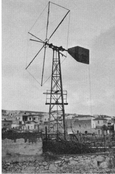
Figure 8. Small water-pumping wind turbine in Eastern Crete with its sail furled during the rainy winter season [2].
