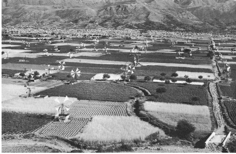
Figure7. “Skimming” the wind for pumping water was practiced using about 10,000 sail-driven small wind turbines during the summer on the Lassithion plateau, Crete [2].
