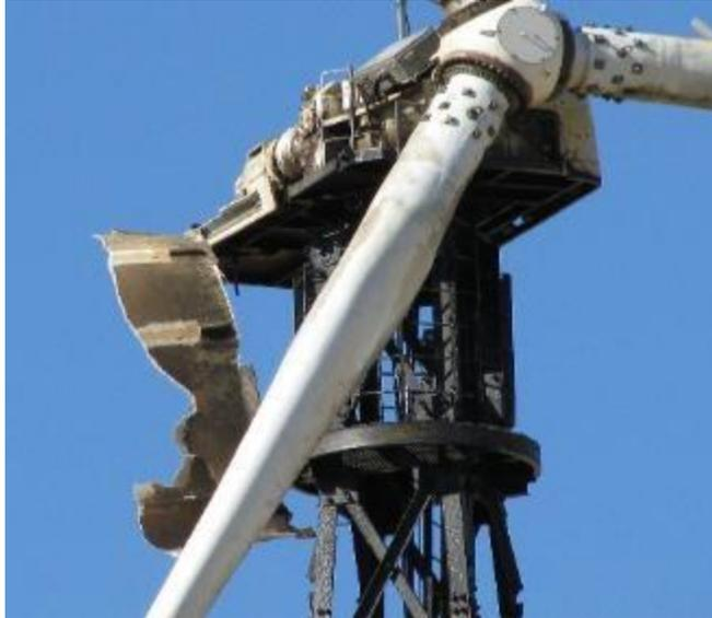
Figure 1. Decaying abandoned truss tower style wind turbine in California.
