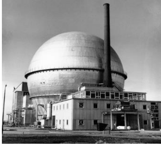
Figure 15. Advanced Gas Cooled (AGR) CO 2 -cooled reactor at Sellafield.
