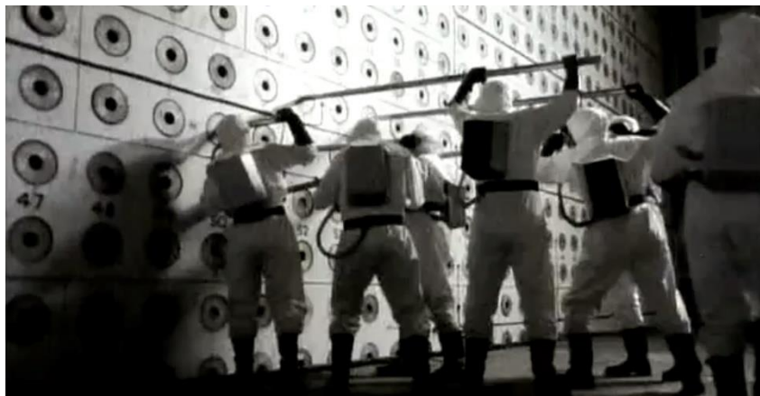
Figure 13. Feeding fuel elements into the Windscale reactors channels.
