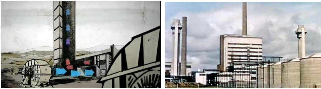
Figure 5. Air circulators and ventilation stacks with filters atop them at the Windscale reactors.
