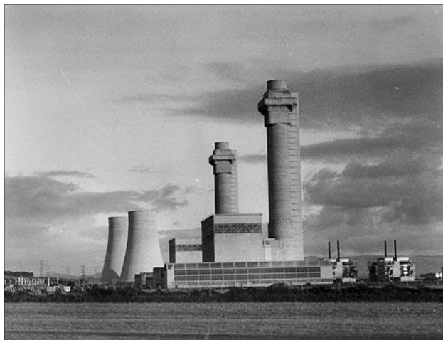
Figure 1. Windscale graphite-moderated air-cooled piles with cooling towers (left) and ventilation stacks (center) with air filters on top,
