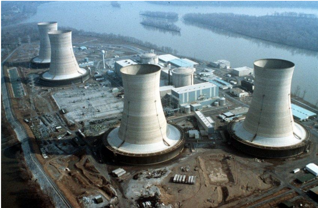
Figure 1. Metropolitan Edison's unit 2 Pressurized Water Reactor (PWR) of 961 MWe of electrical capacity is the capped cylindrical building between its two cooling towers in the foreground. Unit 1 in the back was unaffected by the accident and continued operation.
