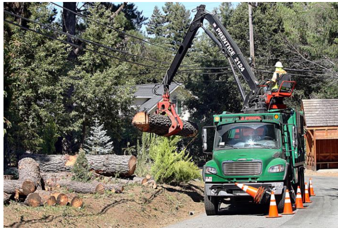
Figure 28. Tree removal around overhead power lines. Santa Cruz, California.
