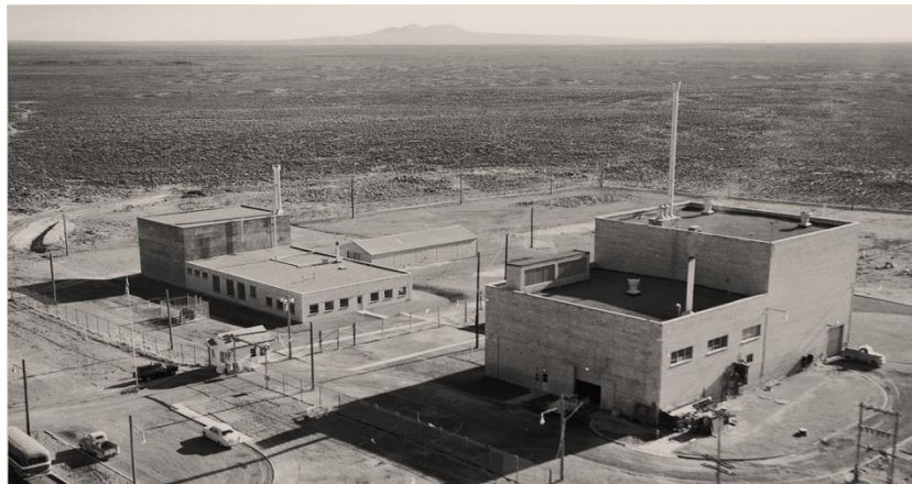
Figure 1. Exterior of Experimental Breeder Reactor, EBR-1 plant.
