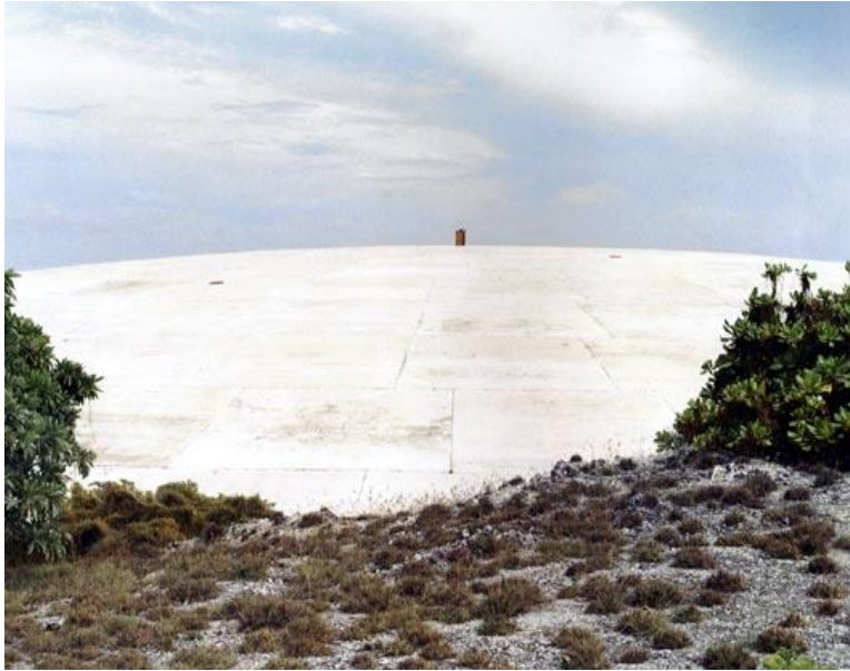
Figure 42. Concrete dome 18 inches in thickness entombs 111,000 cubic yards of contaminated soil and debris on Runit Island. As a prank by bored service-personnel, a red painted barrel on its top makes it visible as a nipple from aircraft flying overhead.
