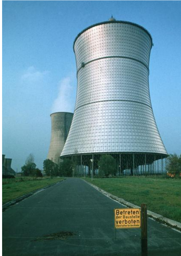
Figure 10. THTR dry cooling tower in the front and water cooling tower in back.
