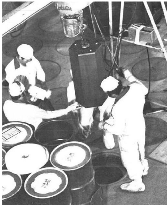
Figure 4. One of 1482 prismatic graphite blocks lowered into the core of the Fort Saint-Vrain HTGR. Photo: General Atomics (GA).
