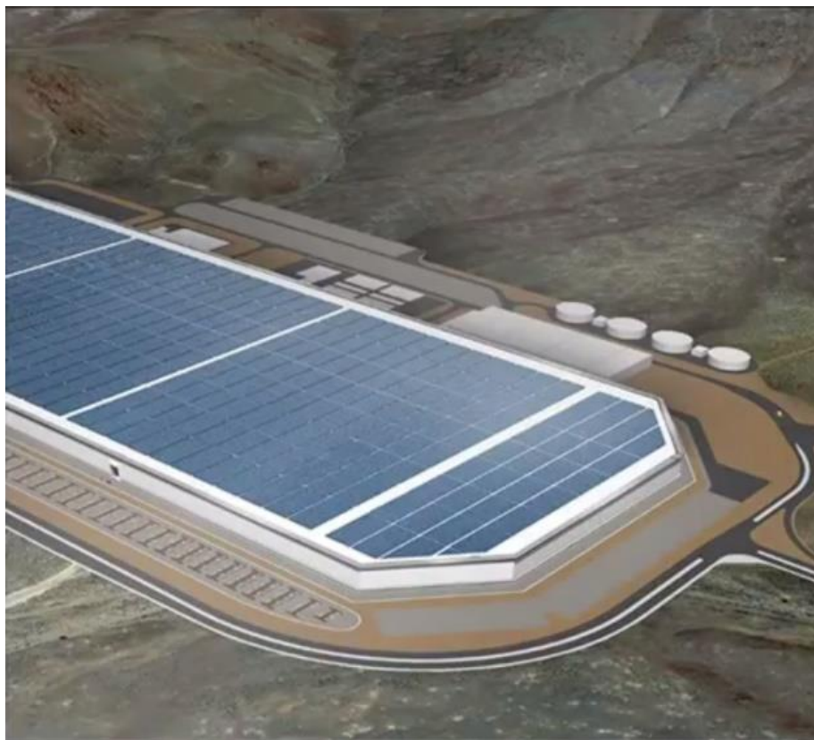
Figure 4. Gigafactory1 solar-powered battery manufacturing facility in Nevada, USA. Source: Tesla Power.
