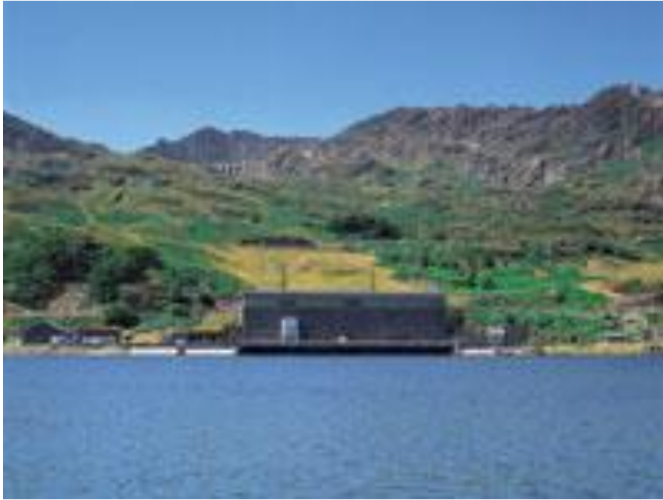
Figure 13. View of the Ffestiniog pumped storage project on Stwlan Dam and Reservoir, UK [4].
