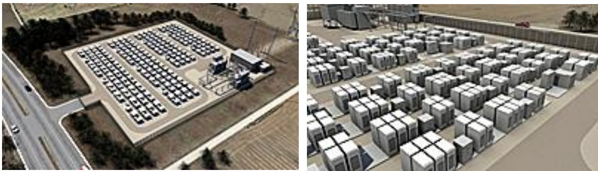
Figure 4. Utility electrical storage configurations. Source: Tesla Power.
