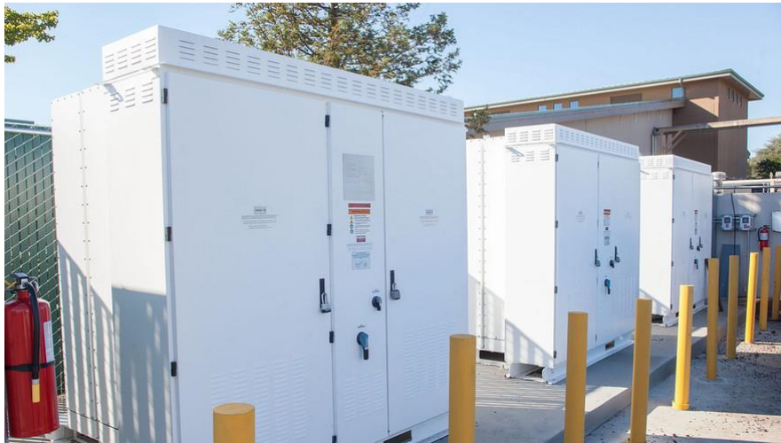
Figure 3. Powerpack units used for refrigeration at Jackson Family wineries in Central and Northern California, USA.
