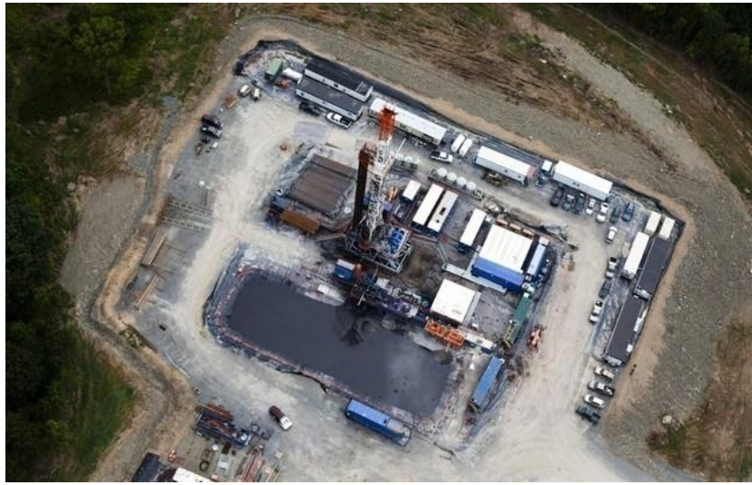
Figure 6. Hydraulic fracturing well site.
