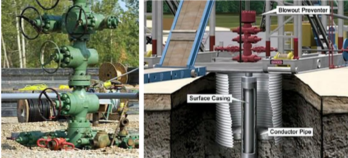
Figure 10. Blowout Preventer (Christmas Tree) and well casing with associated monitoring instrumentation. Source: Royal Shell.
