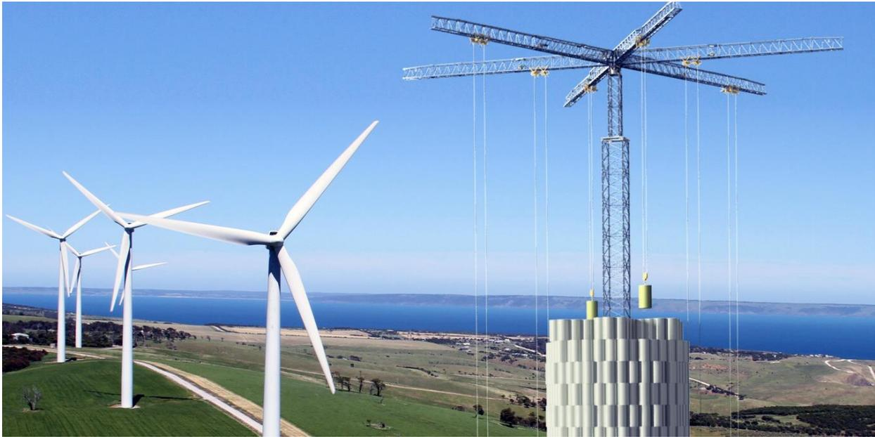
Figure 1. Wind turbines electricity stored then retrieved from a gravitational potential energy storage tower.
