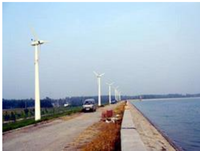
Figure 2. Row of HGenerators 3.4 kW turbines along water shore.
