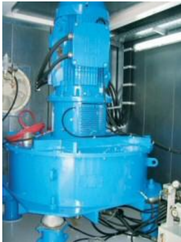
Figure 7. Enercon Flywheel. Source: Enercon.
