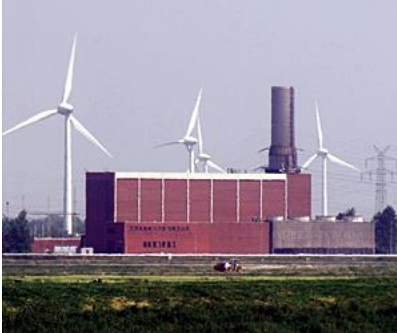
Figure 5. A 290 MW Compressed Air Energy Storage (CAES) in conjunction with wind power at Huntorf, Germany [9].
