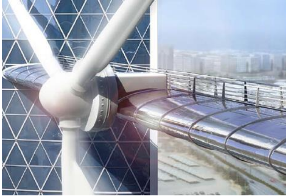
Figure 9. Wind turbine attached to a bridge at the Bahrain World Trade Center.
