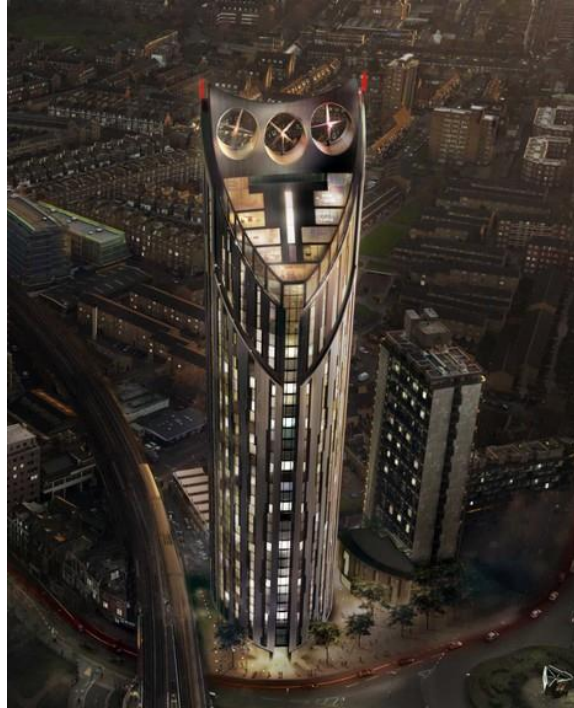
Figure 13. Apartment building at Elephant and Castle in Southwark, London, with three wind turbines integrated into the top of the building.
