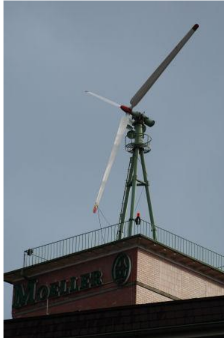
Figure 2. Tied down rotor on an inoperational Allgauer derivative wind turbine on top of a building at Holzhausen, Rheinland-Pfalz, 2005.
