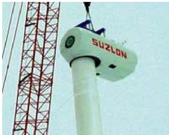
**Fig. 3: Installing nacelle at Minnesota wind park project.**
