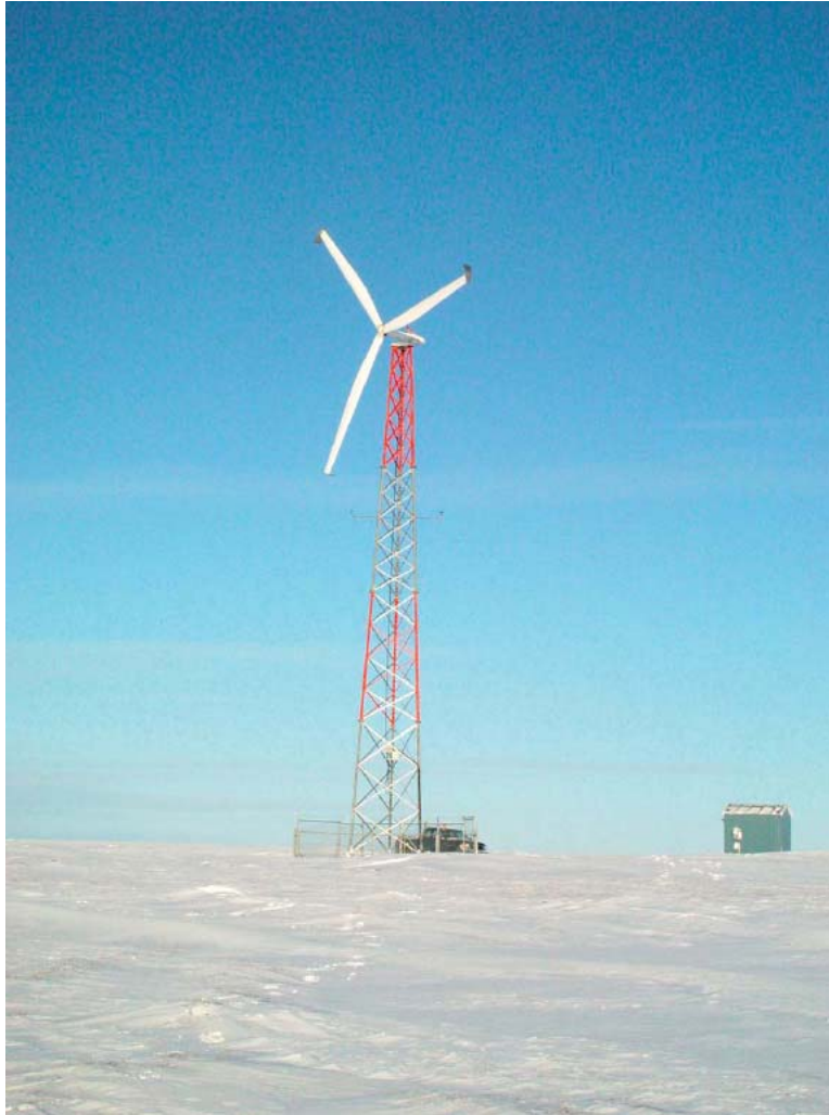
Figure 1. Wind turbine of 50 kW rated power in the arctic harsh environment. Source: Nunavut Wind Corp.
