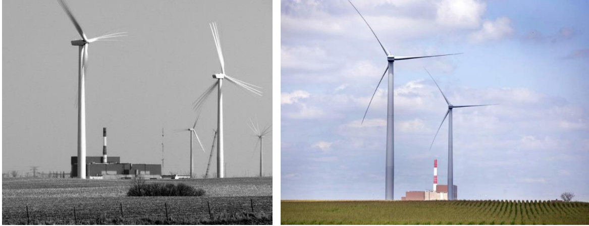
Figure 4. Symbiotic coupling of nuclear and wind technologies views during winter and summer. The two-units 2,309 MWe Boiling Water Reactors, BWRs LaSalle nuclear power plant near Marseilles, Illinois operated by Exelon Nuclear corporation and the Grand Ridge Wind Farm operated by Invenergy LLC in the adjacent farmland near Ransom in Illinois, USA. The nuclear reactor and the wind turbines are both manufactured by the General Electric (GE) Company. The GE 1.5 MW SLE wind turbines have a hub height of 80 m and are net recipients of electrical power from the grid on a standby basis, but then become net exporters of electricity into the electrical grid under favorable wind conditions.
