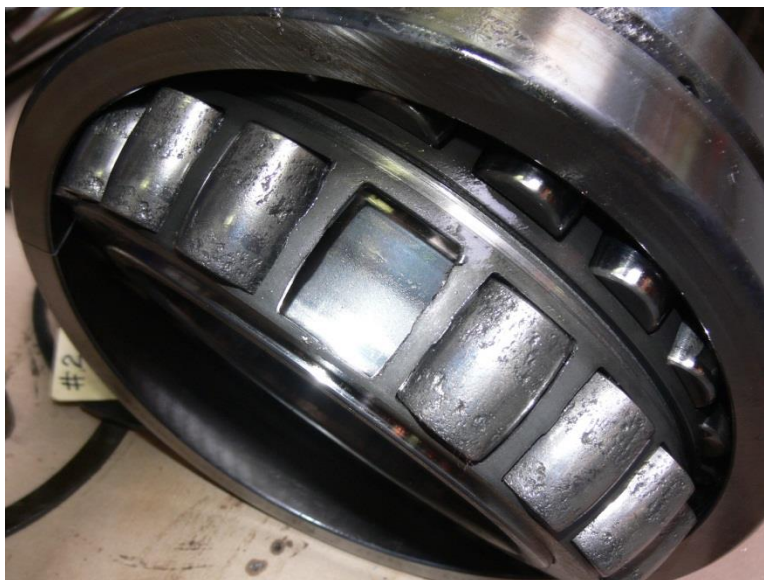
Figure 5. Effect of turbulence and wind wakes on ball bearings of a wind turbine gearbox. Source: NREL.
