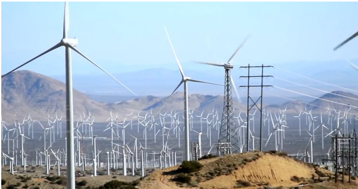
Figure 9. Siting wind parks in the mountain passes of California takes advantage of the tunnel effect.
