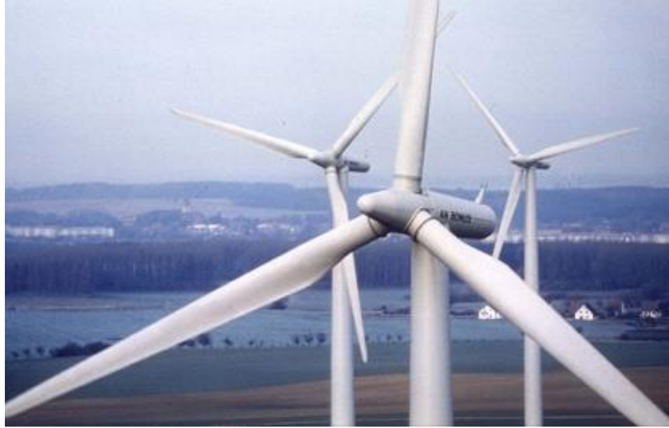
Figure 13. The Ravensburg Krempin wind farm, Germany.
