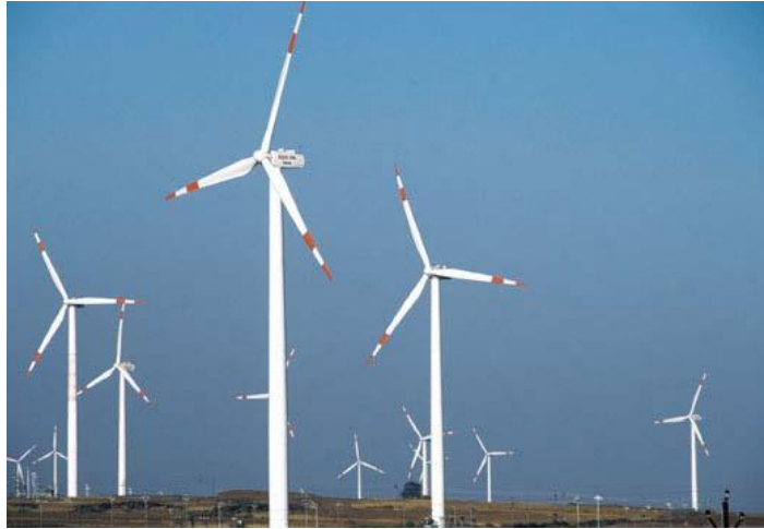
Figure 15. Dhule, India wind-park uses the Suzlon S64-1.25 MW wind turbines. The stripes painted on the rotor blades are intended as a visual warning to flying birds.
