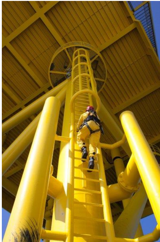
Figure 10. Steel foundation for offshore wind turbine.
