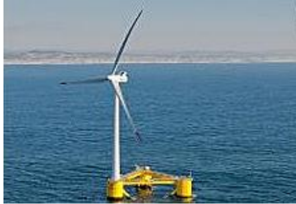
Figure 26. Floating wind turbine at Agucadoura, Portugal.
