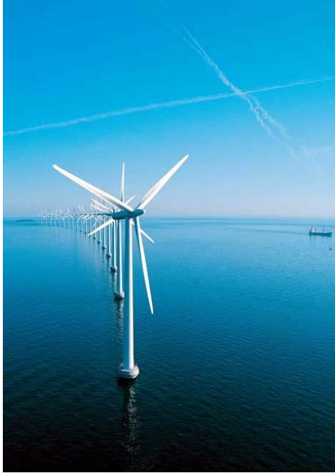
Figure 3. Offshore 40 MW wind farm using 2 MW wind turbines, Denmark. Source: Bonus energy.
