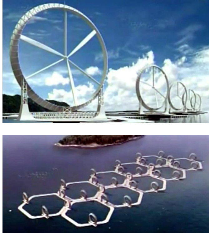
Figure 8. Conceptual floating diffuser wind turbines off the coast of Japan.
