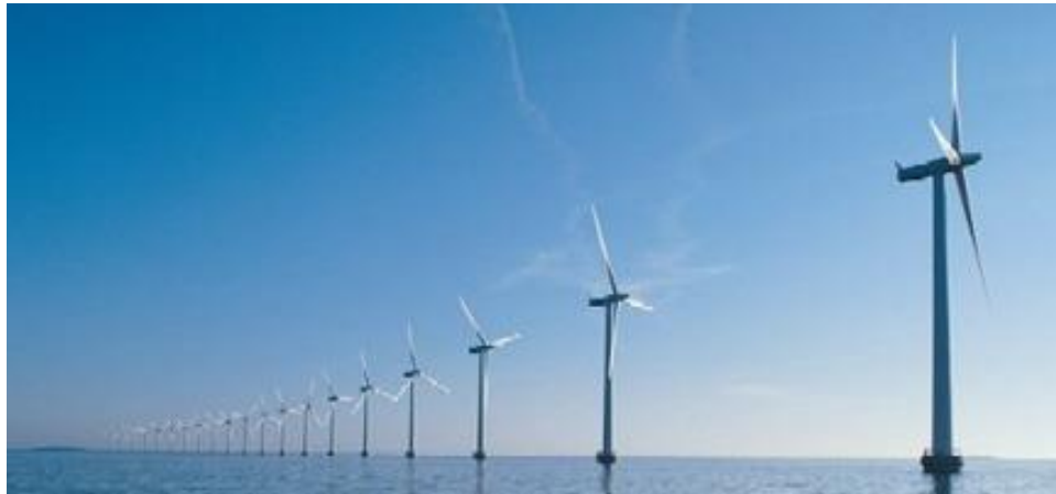
Figure 9. Vindeby, Denmark, first offshore wind farm.
