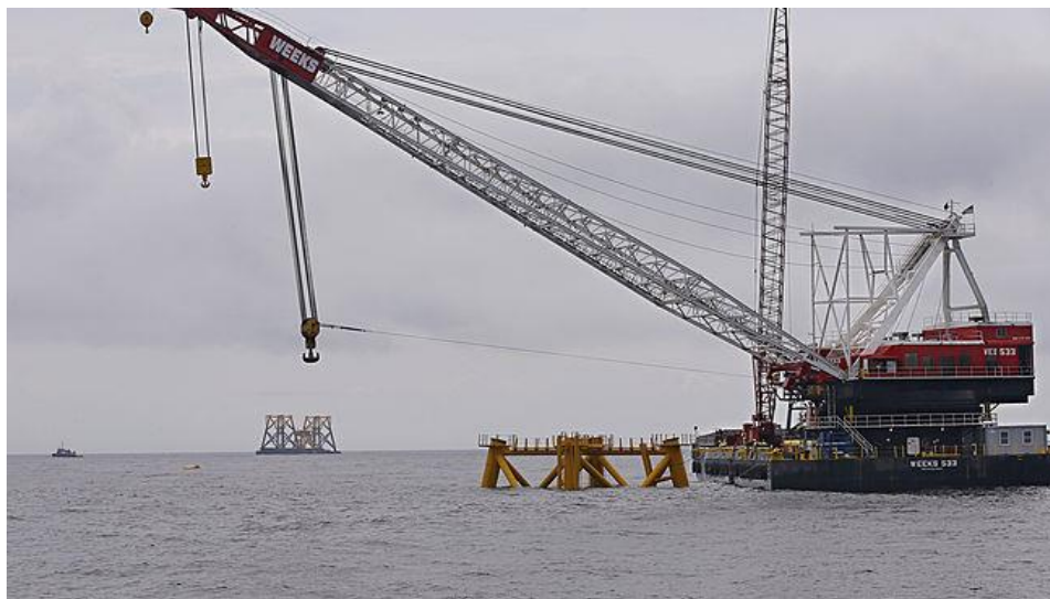
Figure 1. Block Island, Rhode Island offshore wind turbines foundation jackets, July 27, 2015. Source: Deepwater Wind.
