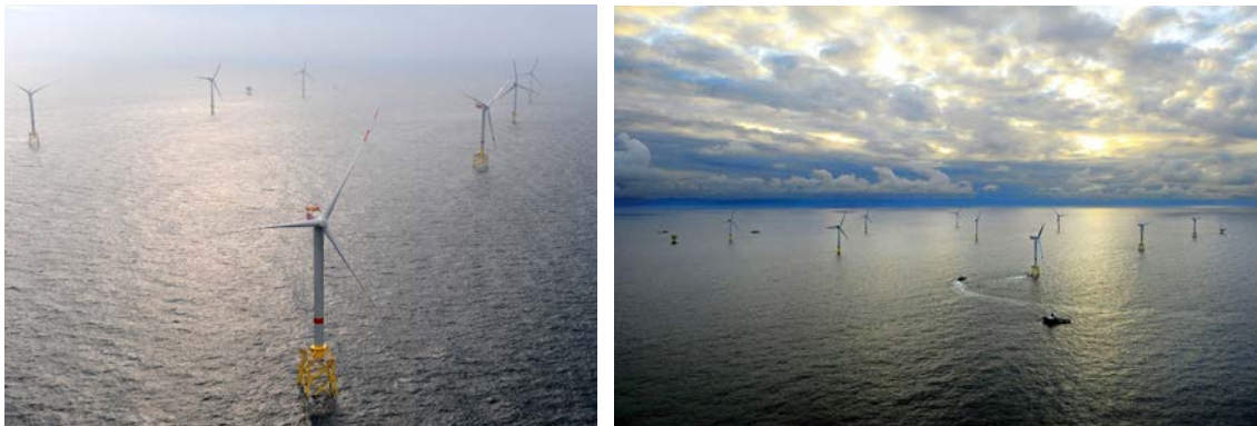
Figure 11. Alpha Ventus offshore wind farm, Germany. Source: DPA.
