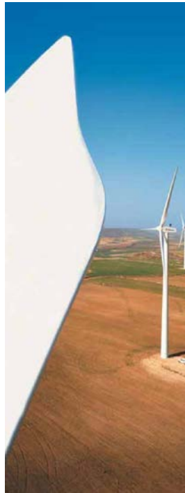
Figure 8. Tapered rotor tip to reduce the noise effect. Source: Gamesa.
