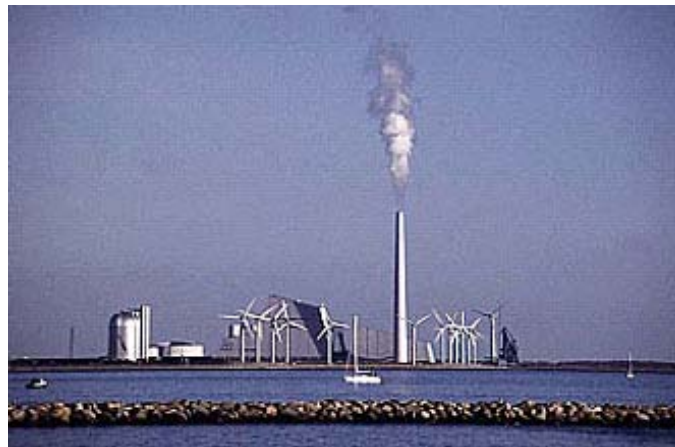
Figure 10. Avedøre wind farm compared with coal fired power station, 5 kilometers from Copenhagen, Denmark.
