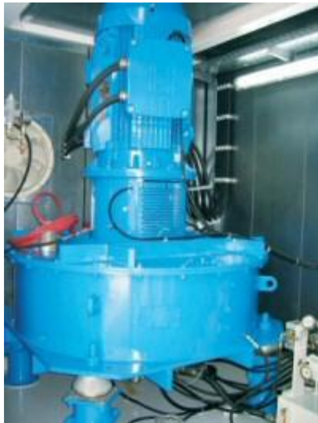
Figure 7. Enercon Flywheel. Source: Enercon.
