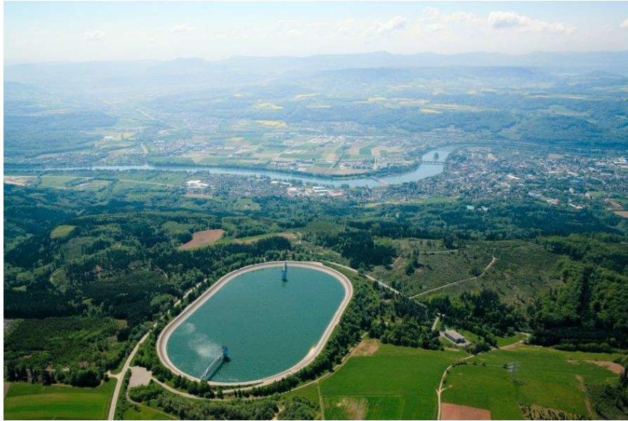
Figure 4. Eggberg reservoir supplies water to the Schluchsee power plant. Schluchseewerg AG Photo.
