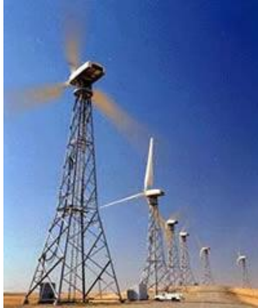
Figure 23. Lattice or truss tower for wind turbines.
