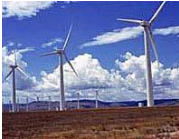
Figure 21. Conical wind machines towers.
