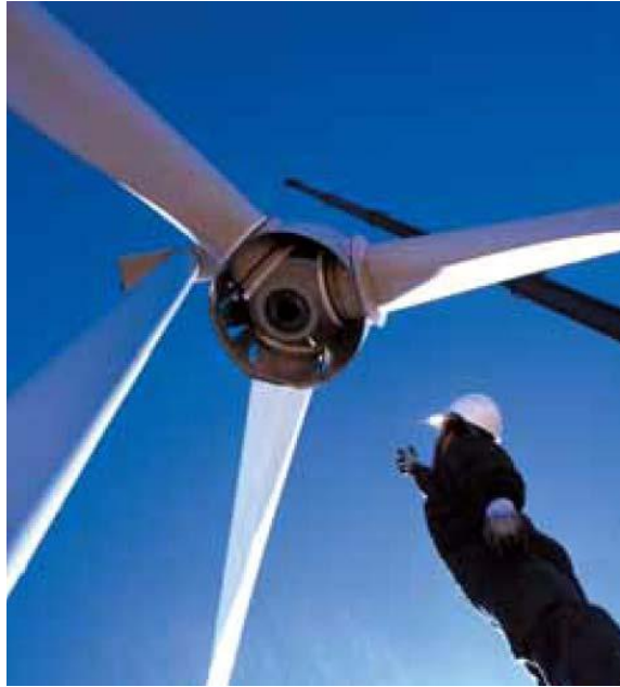
Figure 10. Installation of the hub assembly. Source: Gamesa.
