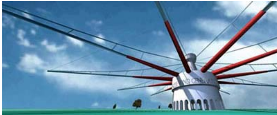
Fig. 7: Carousel kite generator power producing plant.
