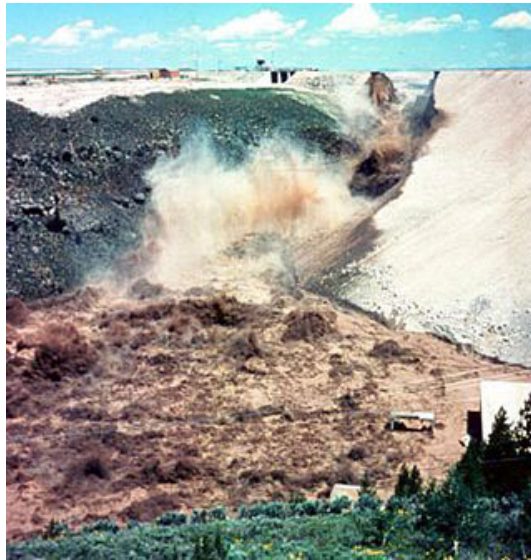
Figure 52. Breach of Teton Dam on June 5, 1976. Photo: Eunice Johnson.
