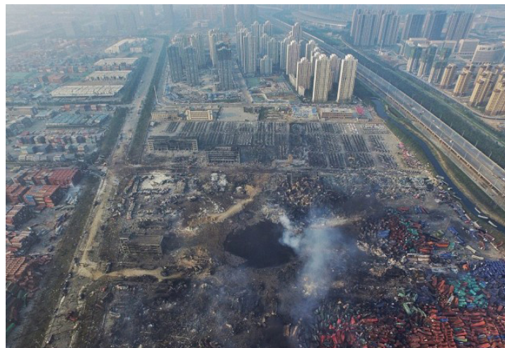
Figure 93. Crater resulting from Tianjin chemical explosions, China.
