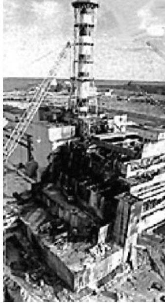
Figure 87. Damaged unit 4 of the Chernobyl plant, before being enclosed in a concrete structure designated as the “sarcophagus.” Accident occurred on April 26, 1986.
