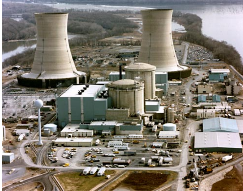
Figure 88. Metropolitan Edison's units 1 and 2 Pressurized Water Reactors (PWR) of 961 MWe electrical capacity each with two cooling towers. An accident occurred at unit number 2 on March 28, 1979, putting it out of service.
