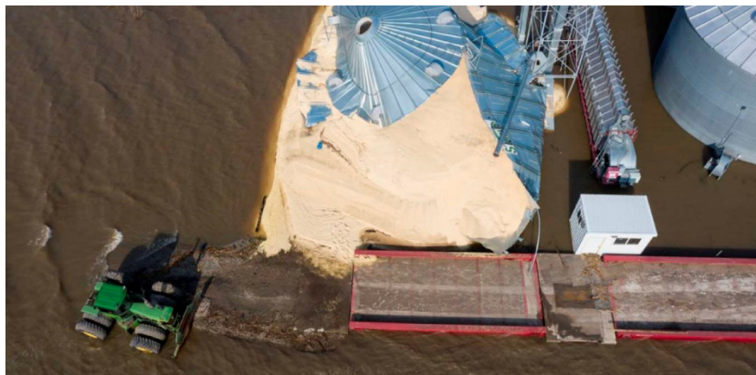
Figure 51. Grain bin collapse due to flooding at Hamburg, Iowa, March 2019. In the Great Flood of 1927, 27,000 square miles were inundated in the USA and one million people were displaced.
