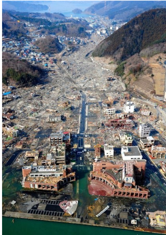
Figure 29. Tsunami damage at Onagawa, March 11, 2011, Japan.
