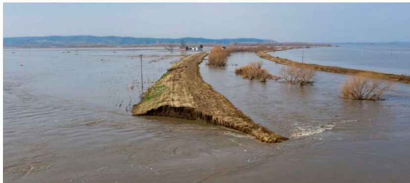
Figure 50. Levee breached on Missouri River near Montescue, Missouri, March 31, 2019. At least 62 levees had been breached or overtopped in the American Midwest in March 2019, and hundreds of miles of levees had sustained damage.
