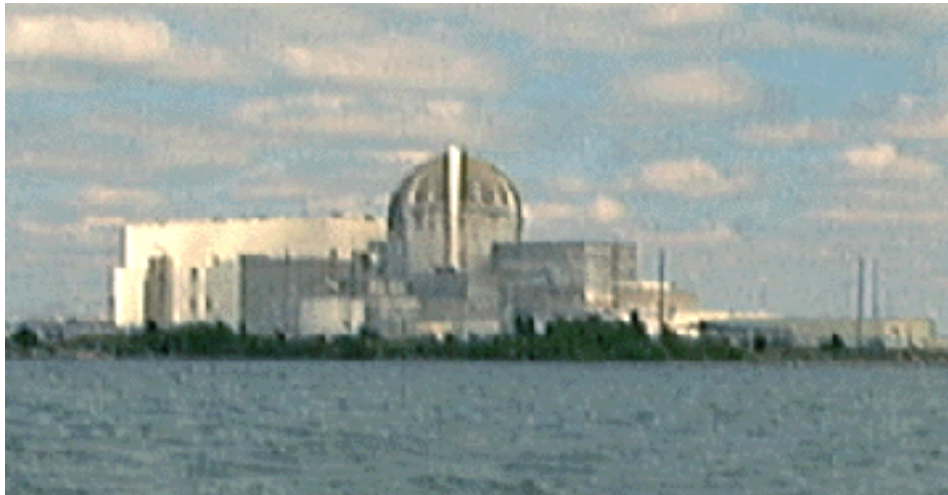
Fig. 5: Cooling lake around Wolf Creek power plant, Burlington, Kansas.
