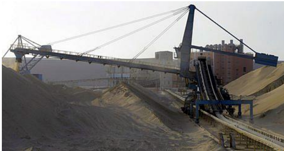
Figure 1. Phosphate ore processing.
