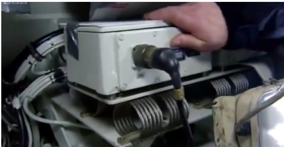
Figure 101. Springs vibration suppression system.
