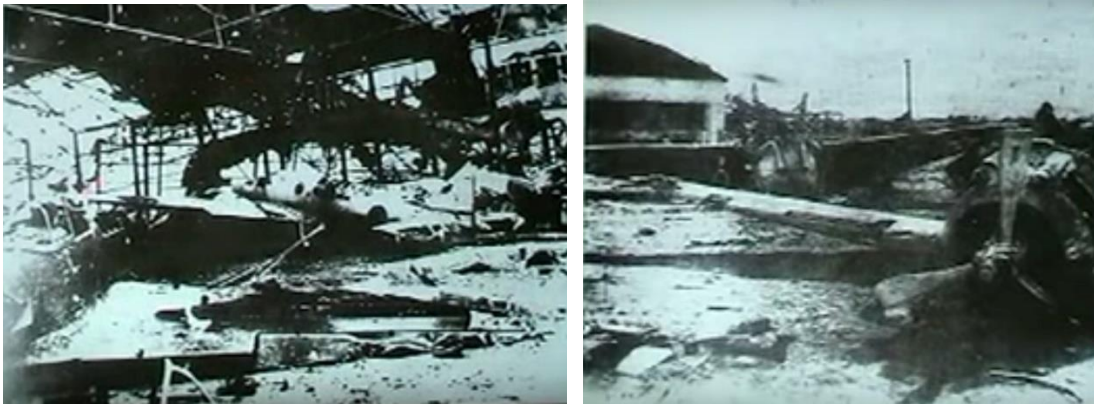
Figure 2. A serious military strike occurred at Clark Field at Manilla, Philippines, 9 hours later on December 8, 1941, where a fleet of B-17 bombers was next targeted and referred to as “McArthur Pearl Harbor.”
