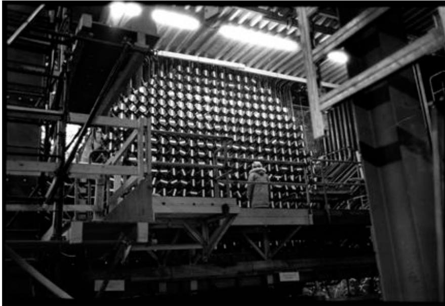
Figure 4. Darlington CANDU reactor face showing the horizontal pressure tubes.
