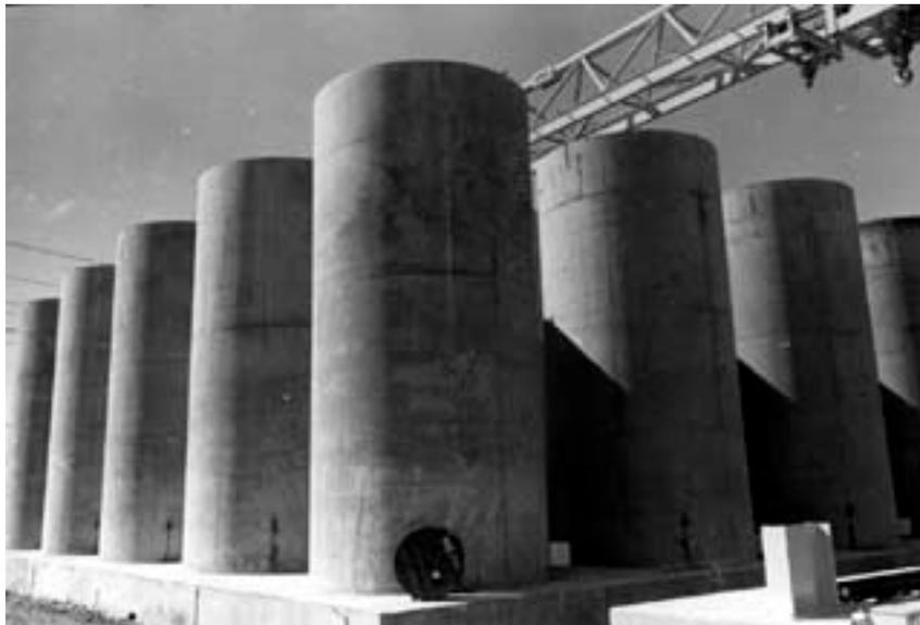
Figure 10. Concrete silos temporarily store the used fuel elements allowing cooling before final recycling or disposal.
