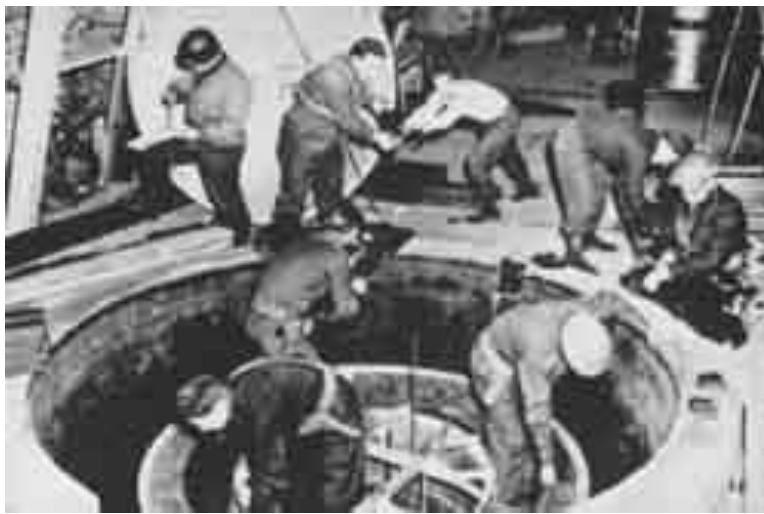
Figure 4. The Alsos team dismantling by hand the heavy water ( D_2O , HDO) subcritical assembly at the village of Haigerloch, Germany.
