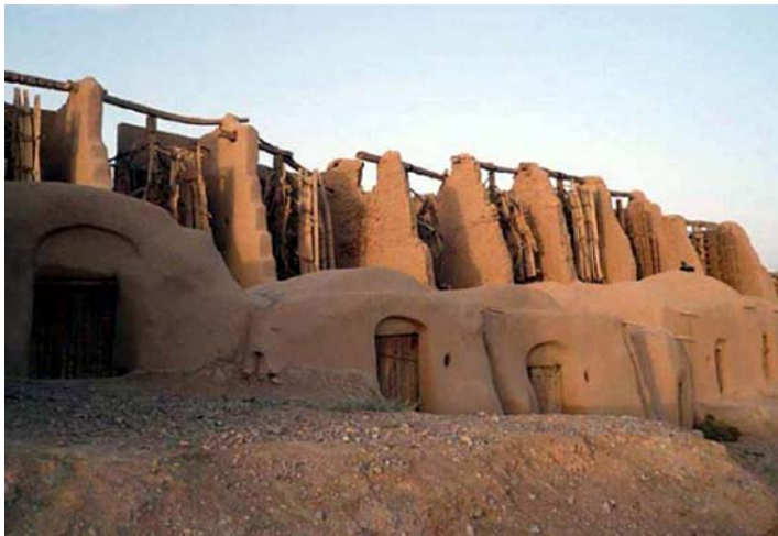
FIGURE 7.3 Remaining vestiges of ancient vertical-axis windmills or “Panemones” at Seistan, near the border between Iran and Afghanistan. The rotors were made from cloth or bundles of reeds and wood.
