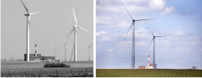
FIGURE 7.10 Symbiotic coupling of nuclear and wind technologies views during winter and summer. The two units 2309 MWe Boiling Water Reactors LaSalle nuclear power plant near Marseilles, Illinois, United States operated by Exelon Nuclear corporation and the Grand Ridge Wind Farm operated by Invenegy LLC in the adjacent farmland near Ransom in Illinois, United States. The nuclear reactor and the wind turbines are both manufactured by the General Electric Company [7].
