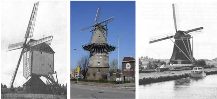
FIGURE 7.7 Evolution of Dutch windmill designs: rotating cage post windmill with rotating lever wheel in the back and pegged wheel acted as a yaw mechanism to rotate the windmill to face the wind (left), tower design (Funenkade Olen windmill, Amsterdam, Holland) (center), and rotating-roof smock design for pumping drainage water (right).
