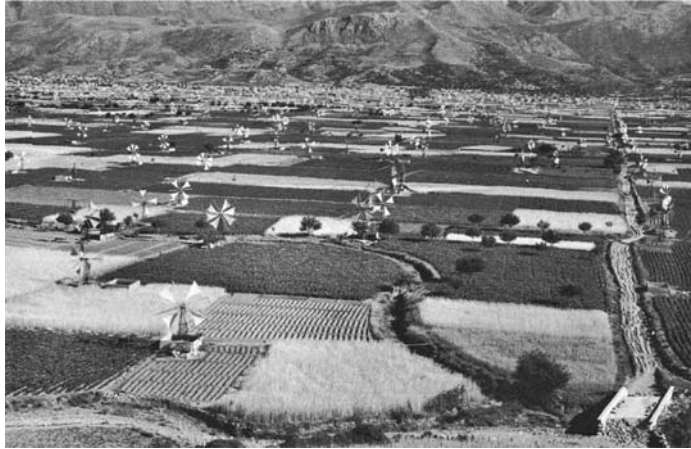
FIGURE 7.5 Sail water-pumping windmills harvesting the wind in large numbers on the island of Crete in the Mediterranean Sea.
