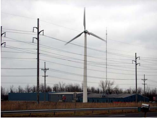
FIGURE 25.1 Single wind turbine providing power to a small business, despite the availability of an electrical grid supply at Rochester, New York: Harbeck Plastics, Inc. It can extract energy from the grid, overcoming the intermittence of the wind and its surplus production; if not stored, can be wheeled into the electrical grid. Courtesy Chris Kabureck.
